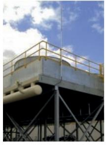
Insulated arrester system in an explosion-prone area
